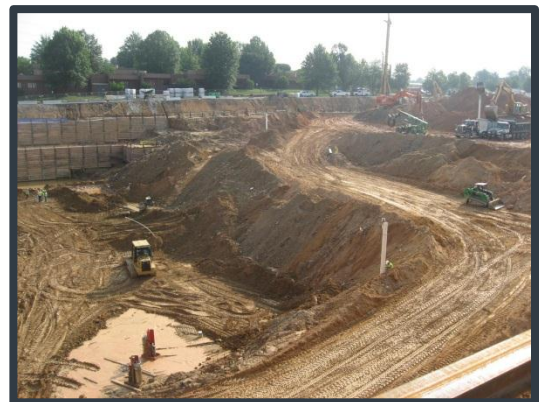
Figure 8: Excavation Ramp
