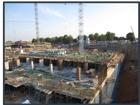
Figure 6: Concrete Slab Construction
