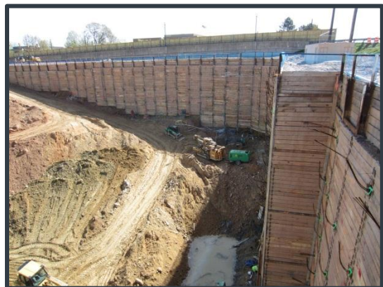
Figure 7: Soldier Piles and Lagging
